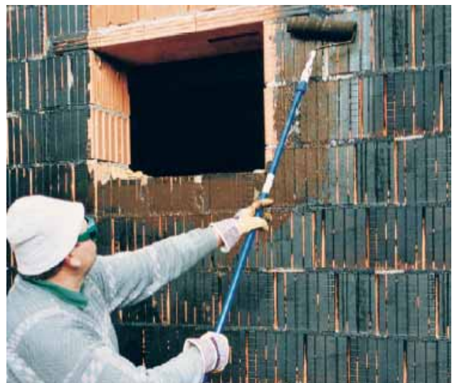
PCI Pecimor F, diluted 1 : 5 with water, acting as a primer for the tanking of structures with polymer-modified thick bitumen coating in accordance with DIN 18 195.
