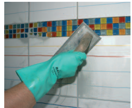
Good workability of PCI Nanofug independent from temperature.
